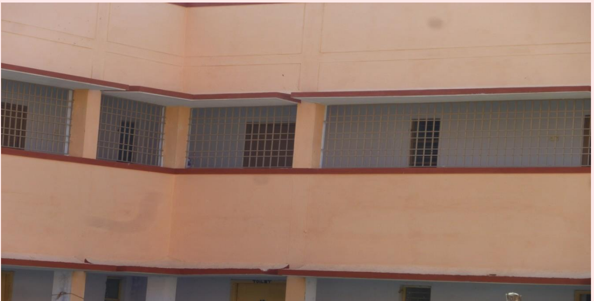
Newly constructed first floor
